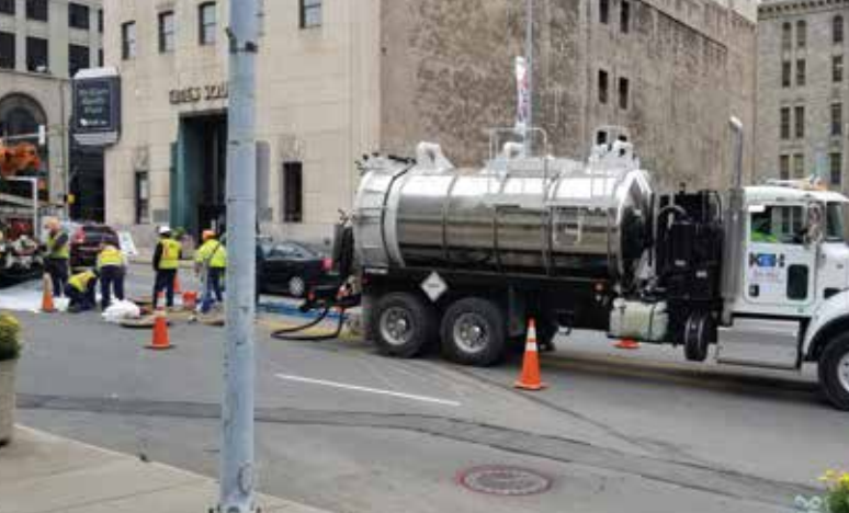
KBHE, Industrial Electric, and Subway Divisions working together to remove existing cable from former oil-filled line on Exchange Boulevard
