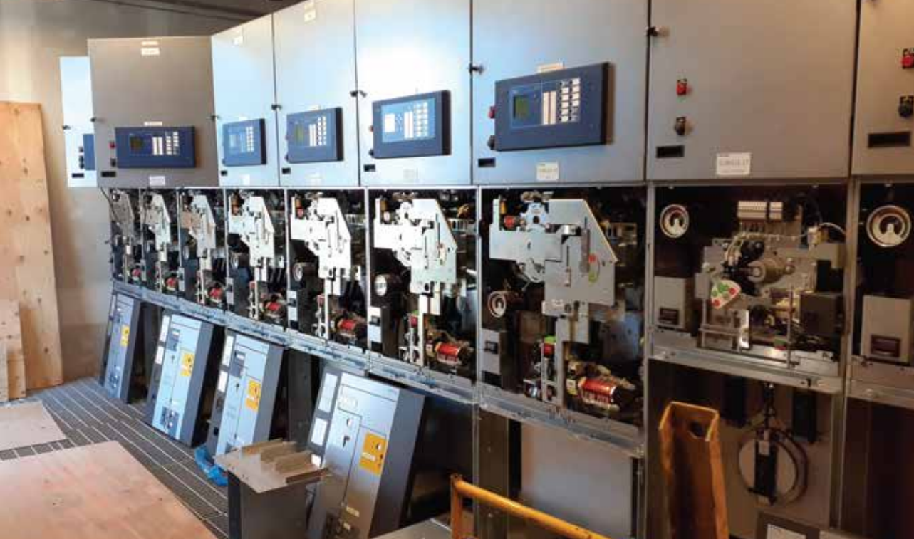
Breakers that open and close circuits that feed the distribution lines in Station 49 on North Goodman Street in Rochester
