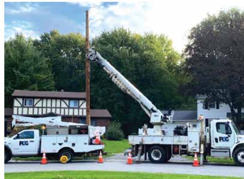
The Street Lighting Division replaces a utility pole in the town of Greece.
