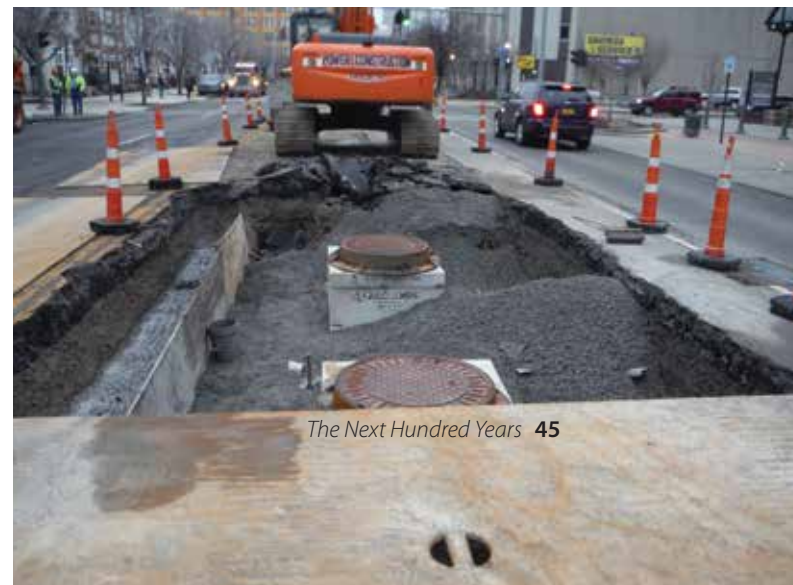
Manholes are installed on Plymouth Avenue for Project 943/944.
