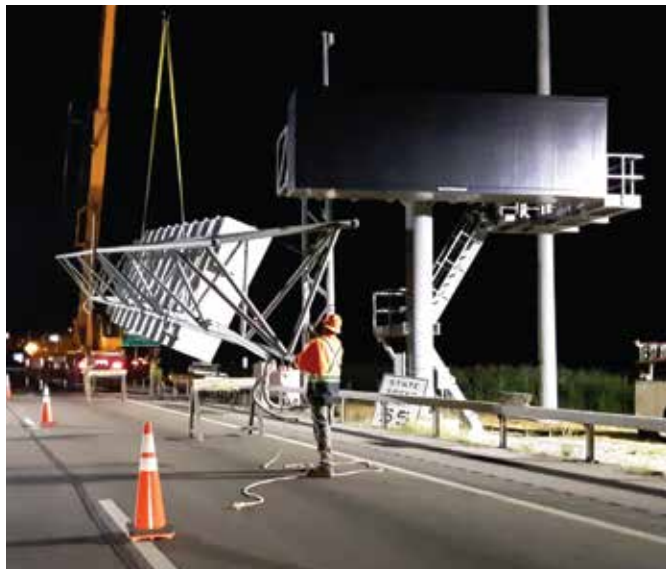
The Signalization Division replaced failing support structures for variable messaging signs on the New York State Thruway in 2019.
