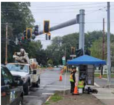
Signalization employees wire a new DOT traffic signal controller to turn on the lights in Watkins Glen, N.Y.
