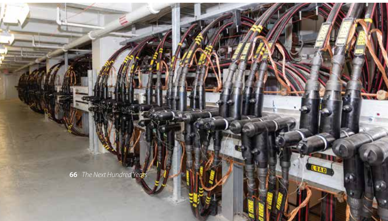
John Roukous and his crew built deadbreak assemblies in Station 38 on Swan Street in Rochester.
