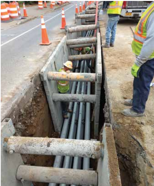
The team installs a 12-way duct bank on Mount Hope Avenue.
