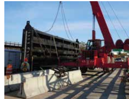
At the Central Avenue Dam, the new gate is lowered into place.
