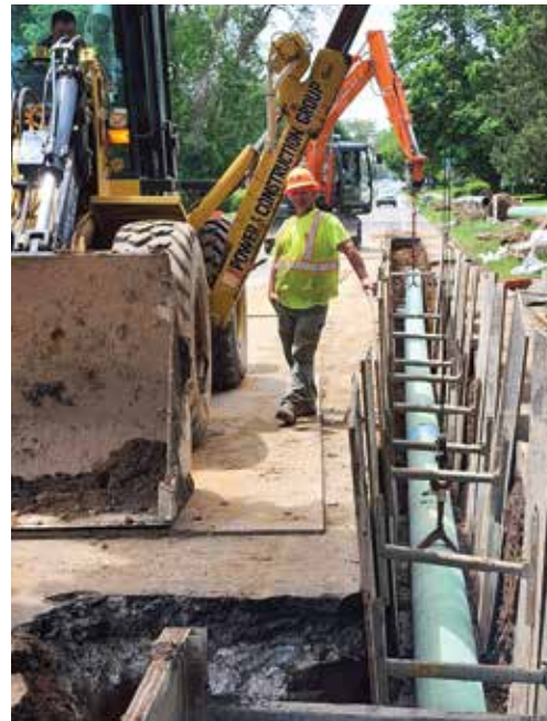
Joe Rodak looks on as the pipe is welded into the main line inside the shoring box on Winton Road.
