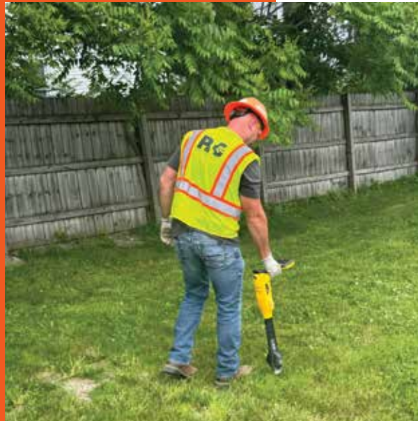
Mark Ditzel locating a ground fault in Greece, N.Y.
