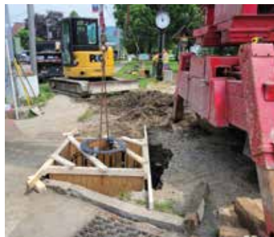
The foundation for a new traffic signal pole and mast arm is set in Watkins Glen.
