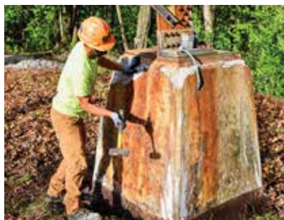
Steven Baxter inspects the concrete footer of a tower by tapping the concrete. If it’s hollow, it is chipped out and replaced.
