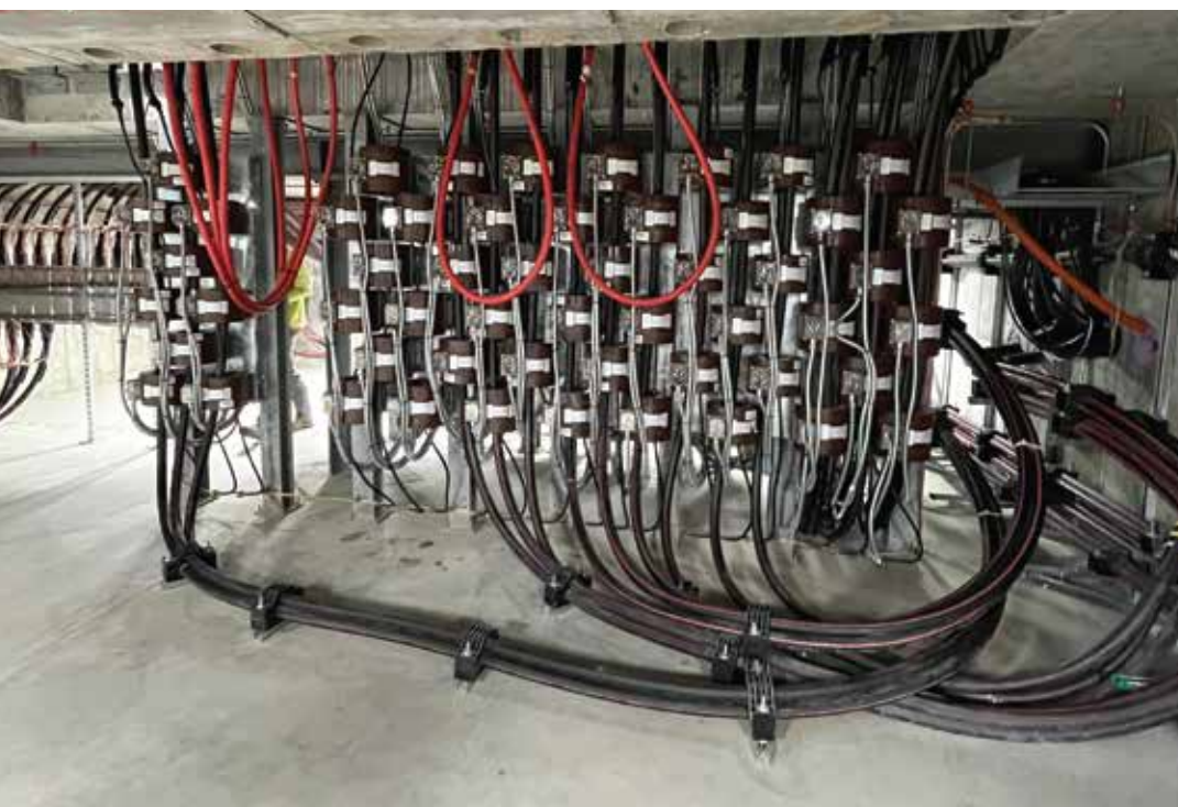
Current transformers (CTs) and medium-voltage cables installed in Station 46 on Ridge Road West in Greece
