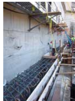
Rebar and forms for concrete are placed at Station 5.
