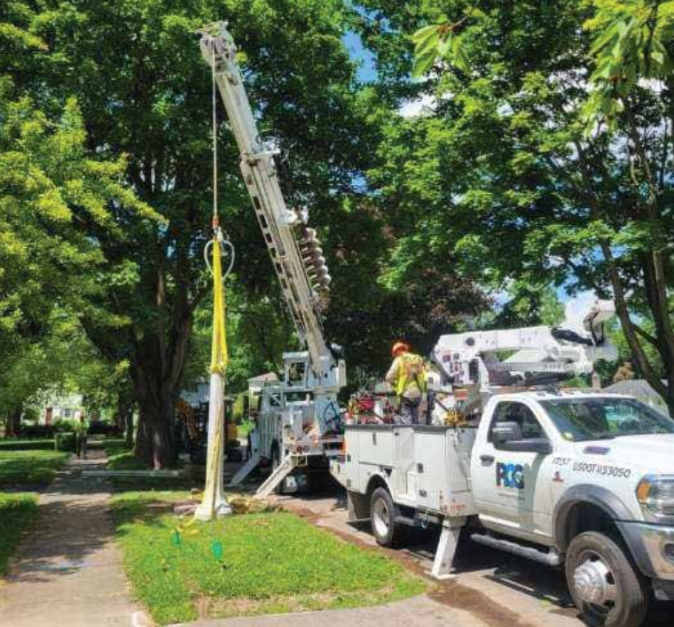
P&CG replaced 100-year-old poles and fixtures for the town of Brighton, N.Y., with replicas in June 2025. Aaron Way prepares a new fixture for installation as the old pole is removed.
