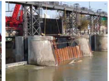
At the Central Avenue Dam, the new gate is lowered into place.
