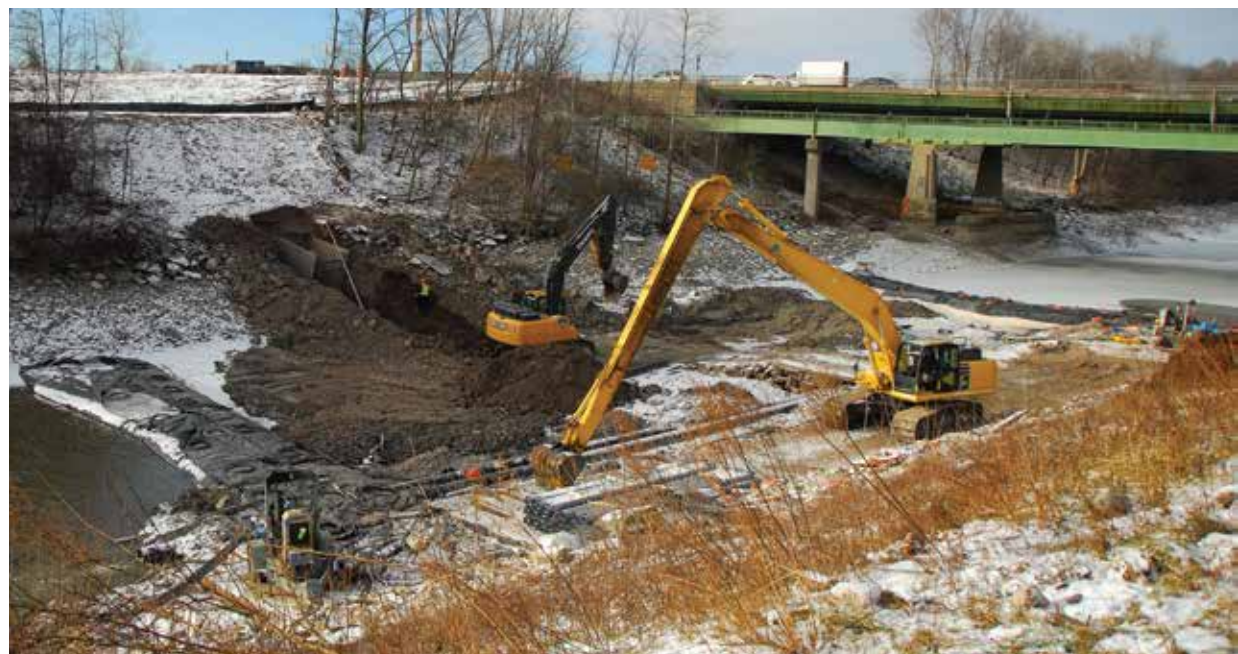
The team excavates through the canal for the final phase of installing the duct bank.
