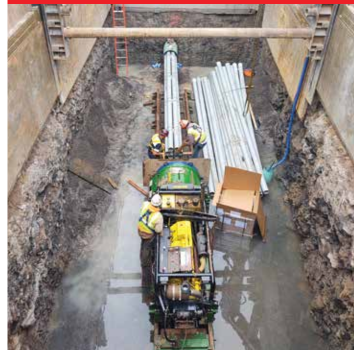
Turner Underground prepares for a large-diameter rock bore over 30 feet deep at the intersection of Plymouth Avenue and Ford Street—part of the Subway Division's 2020 Circuit 806 conduit installation project.
