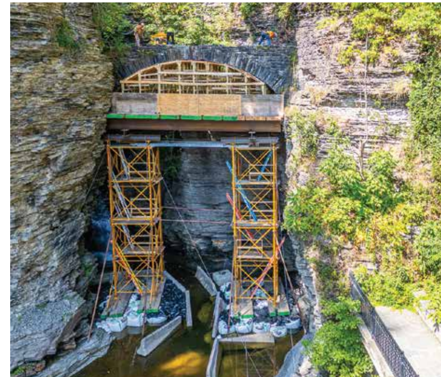
Shoring towers and cribbing support the concrete structure during demolition.
